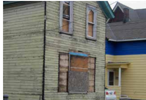
Abandoned and boarded-up home
