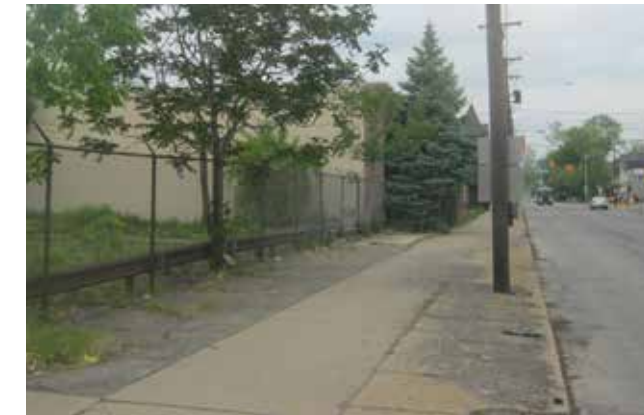
Area within Tremont neighborhood that has insufficient curb heights, and a chain-link fence as an edge treatment.
