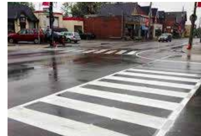
Painted ladder crosswalks are considered high-contrast and are more visible to vehicles
