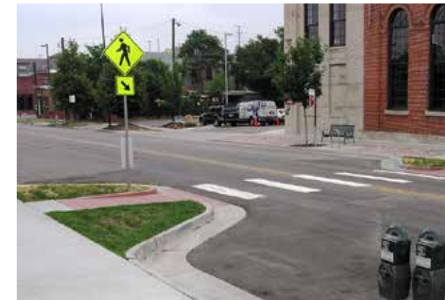
Bulbouts reduce the crossing distance for pedestrians
