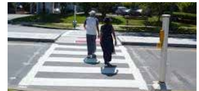
Example of a high-contrast ladder crosswalk with a median pedestrian refuge and a rectangular, rapid flashing beacon, (RRFB)
