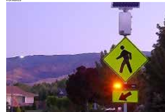
Rectangular Rapid Flashing Beacon
