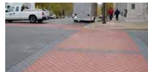
Example of an enhanced crosswalk with colored, stamped concrete.
