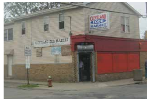
Existing windows have been boarded along the sidewalk, which reduces safety.
