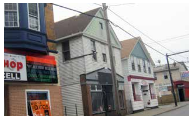
The Stockyard neighborhood has good small scale commercial building stock.
