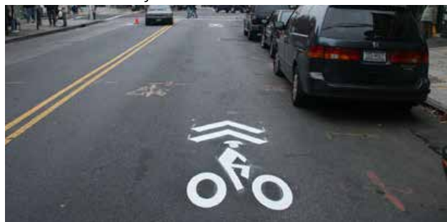
Sharrow markings are recommended from W. 16th Street to W. 65th Street.
